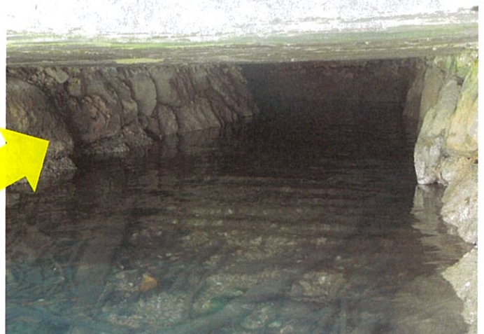
Inside the storm drain.
